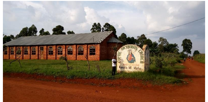
View of the Coptic Church building
